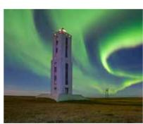
The lighthouse was built in 1938 -1939, the first in Iceland to be built out of reinforced concrete. The lighthouse is the tallest building in South Iceland, 26,2 meters (86 feet) high. It was designed by the engineer Axel Sveinsson as a blend of functionalism and art nouveau (jugendstil). Knarrarósviti lighthouse is part of the beautiful South Coast Lighthouse trail. **GPS** N63° 55′ 28.731″, W20° 40′ 19.063″
